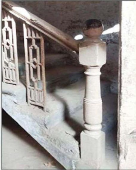
Adamjee building main staircase railing. (Fig 1.1)
