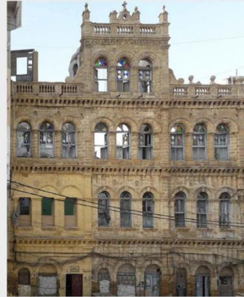
Kanji Building (Fig 1.1)
