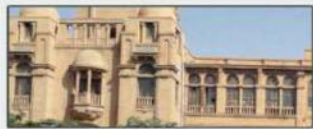
KMC Building (Fig 1.3)
