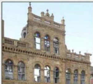
Kanji building (Fig 1.5)
