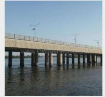
2. Native Jetty Bridge
