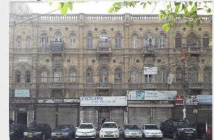
Essajee Ibrahimjee Building (Fig. 1.2)
