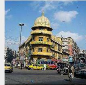
5. Jamshed Katak Building
