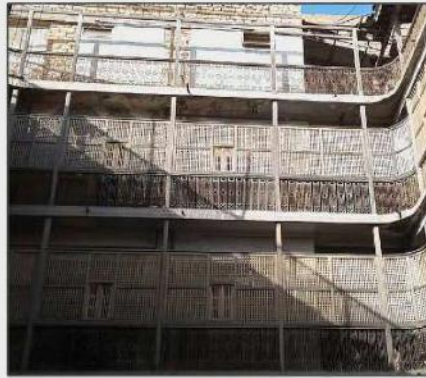
Adamjee Building (Fig 1.2)
