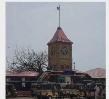
6. Sydenham Passenger Pavilion
