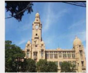
2. Karachi Municipal Cooperation Building
