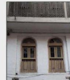
Adamjee building, Grill on the outer side (Fig 1.6)
