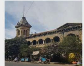
4. Jehangir Kothari Building
