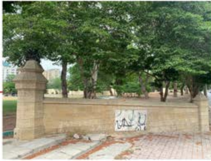
Wall (i') 16' x 9" Intact
