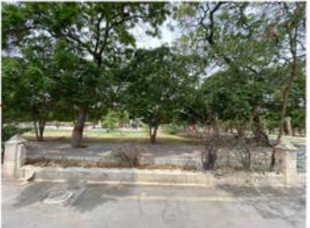
Fence (f) 24' x 4 1/2" Missing
