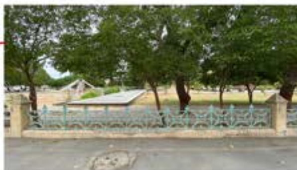
Fence (l) 28' x 8" Intact
