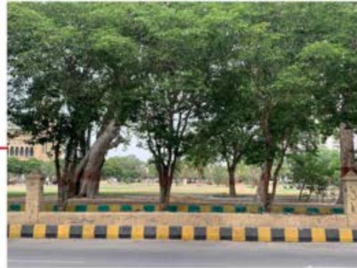
Fence (f) 24' x 10" Missing
