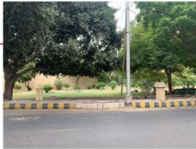
Fence (z) 24' x 3" Missing
