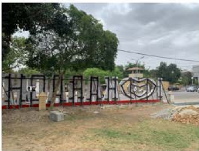
Fence (b') 31' x 0" Missing
