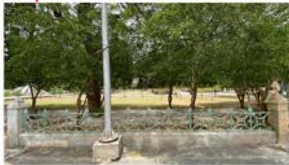
Fence (j) 28' x 8" Intact
