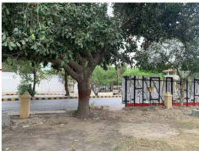
Fence (a') 24' x 5" Missing
