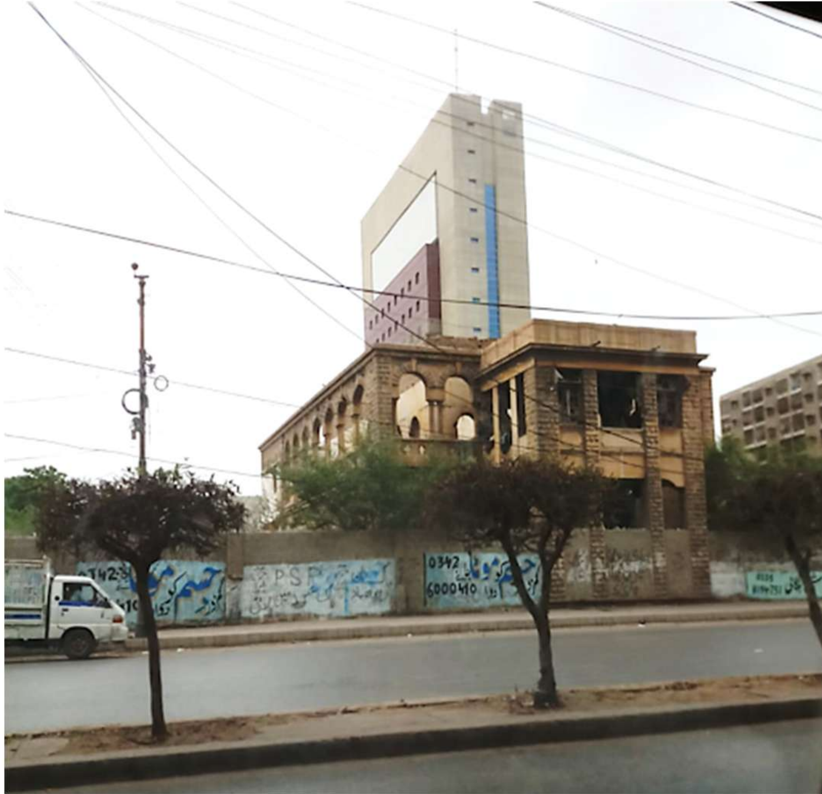
Image 1.0: The verticality can be clearly observed through this image where the high rise building sits atop the decaying heritage building making it seem isolated and neglected. It serves as a reflection of the increasing urban sprawl mentioned above. Photo by Marvi Mazhar (M.A. Jinnah Road).
