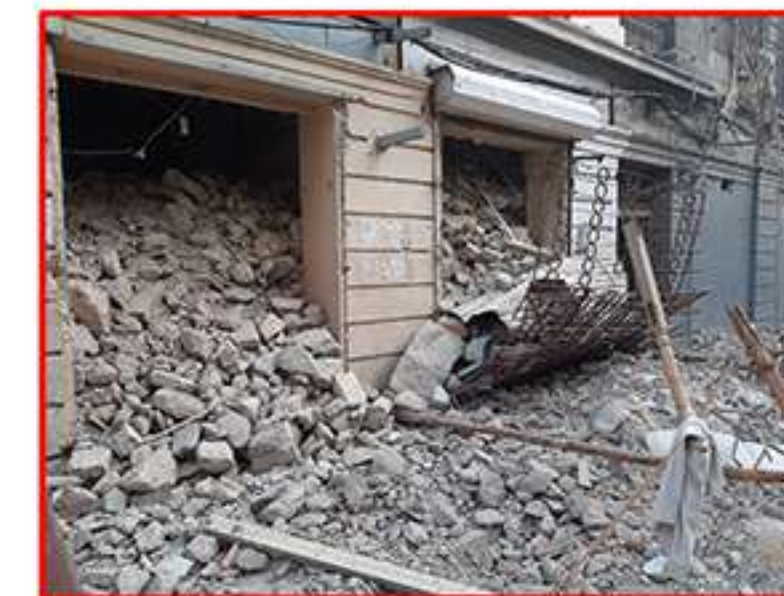
Demolition of Bhattia Bhawan
