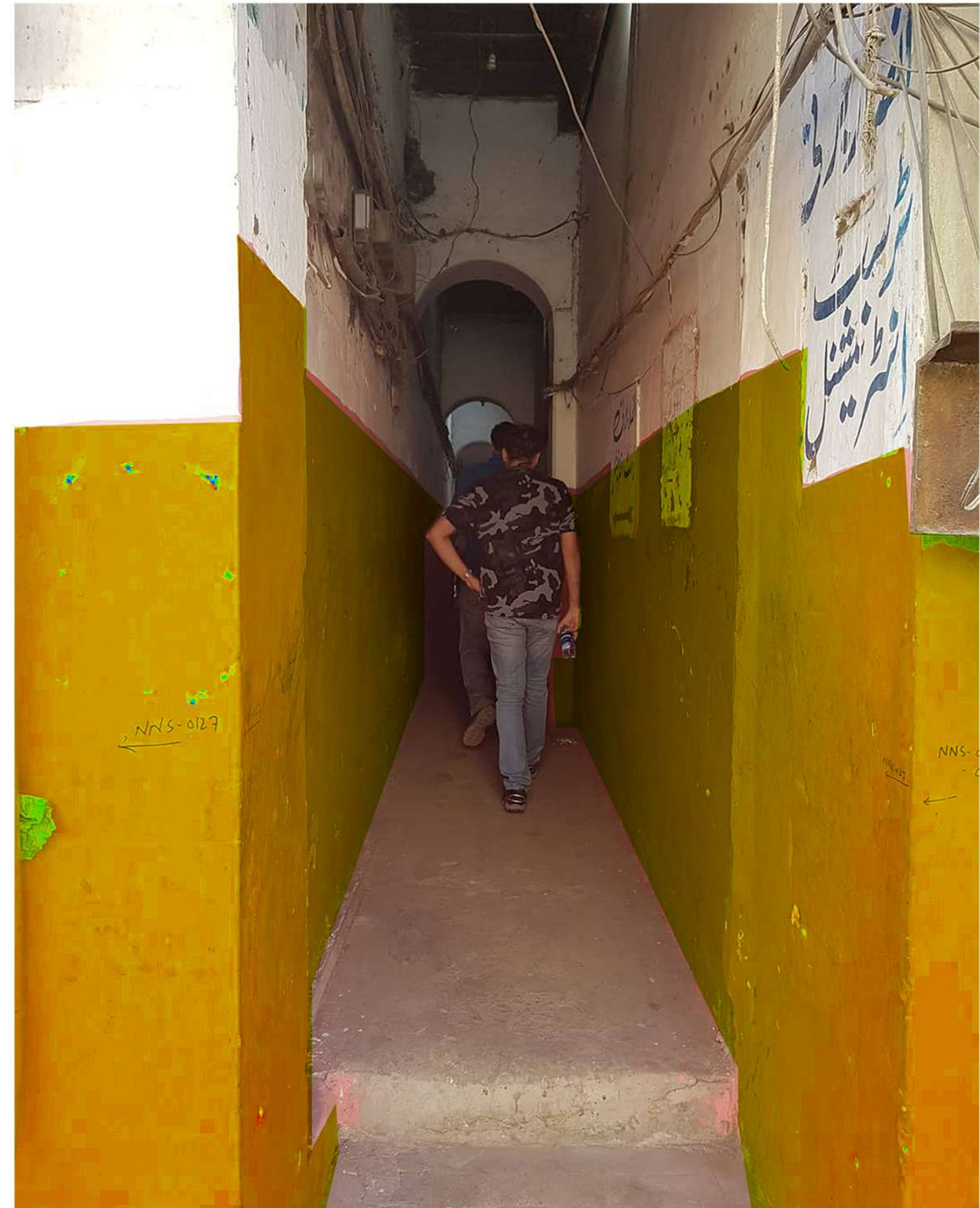
Narrow passageway of Pre-partition building, Hasan Building
