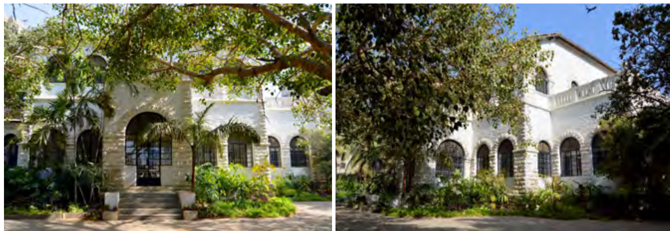
Left: Back Elevation / Right: North-West View Image Copyright of Marvi Mazhar and Associates
