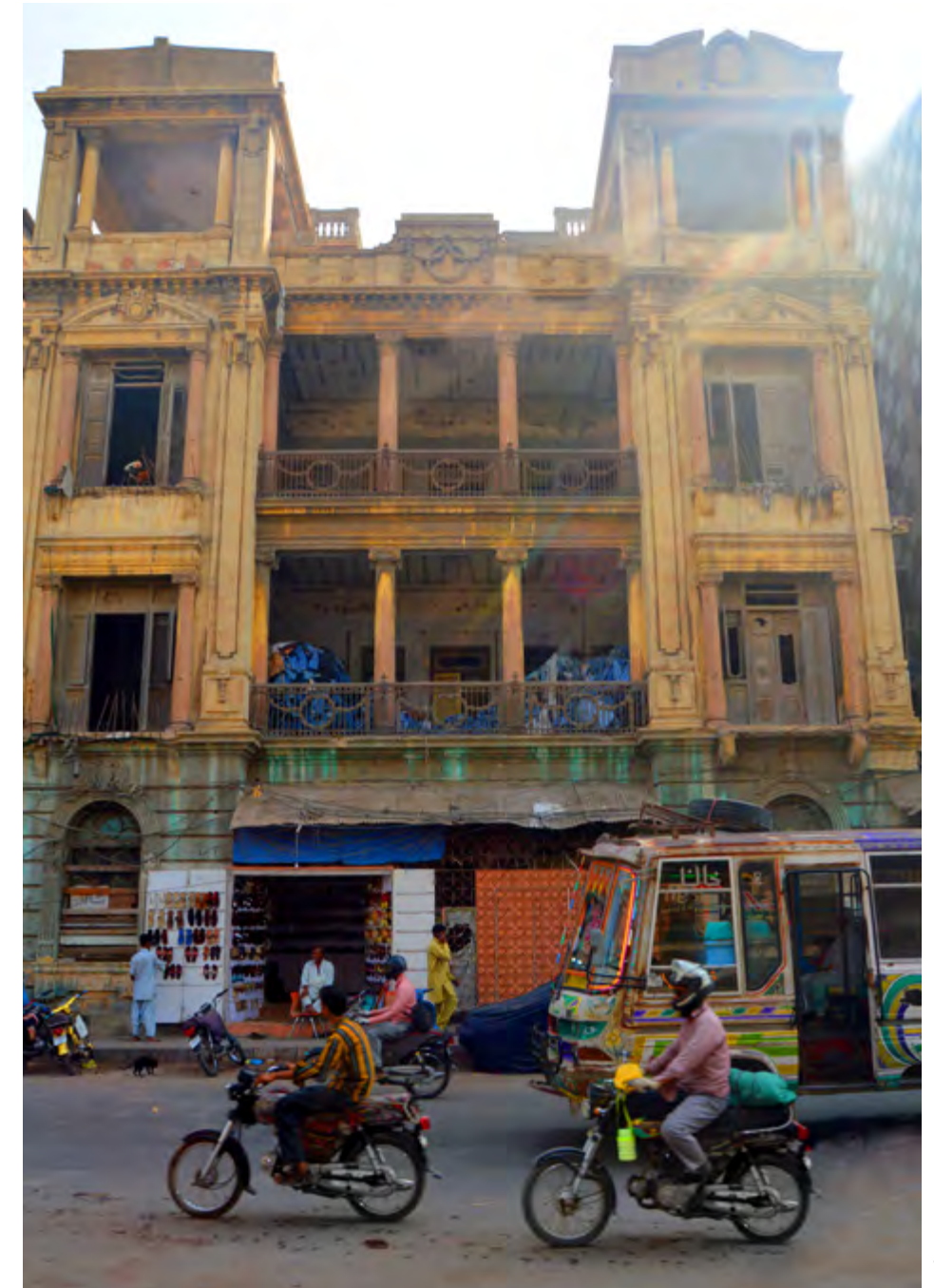
Elevation from Mohammed Bin Qasim Road Image Copyright of Marvi Mazhar and Associates
