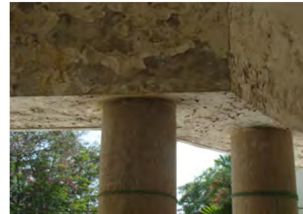
Top Left: Column detail / Centre Left: Documented Flooring / Bottom Left: Entrance with ramp Images Copyright of Marvi Mazhar and Associates
