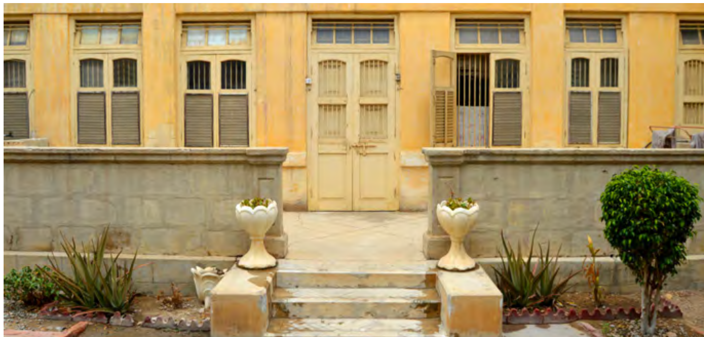
32 Part elevation: Steps to the patio Image Copyright of Marvi Mazhar and Associates
