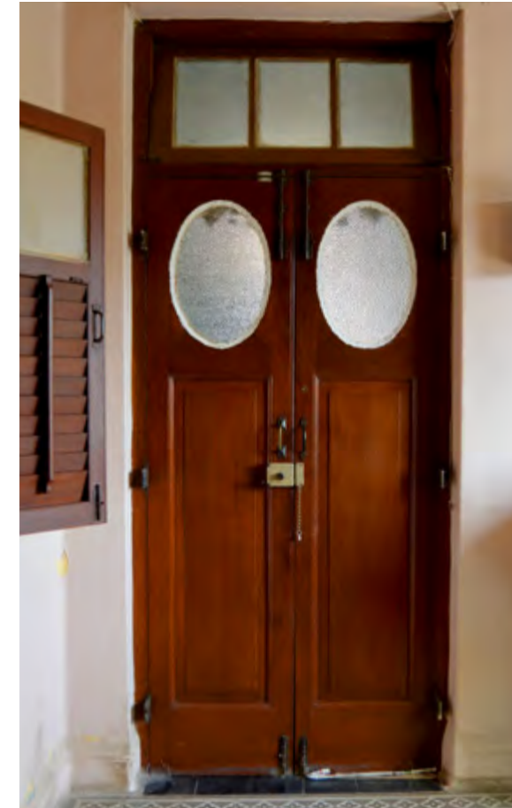
Two panel door with circular glass pane/Ventilator with glass pane. Image Copyright of Marvi Mazhar and Associates
