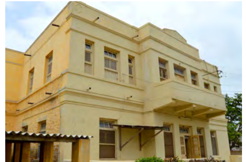
Top: North East View / Centre: Mosaic tile with inlay technique / Bottom: Wooden Staircase, railing and wooden divider with four glass panes Image Copyright of Marvi Mazhar and Associates
