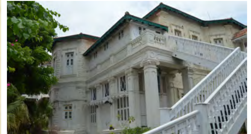
Top: Outdoor staircase to first floor / Centre: Ceramic Tiles / Bottom: South Elevation Image Copyright of Marvi Mazhar and Associates
