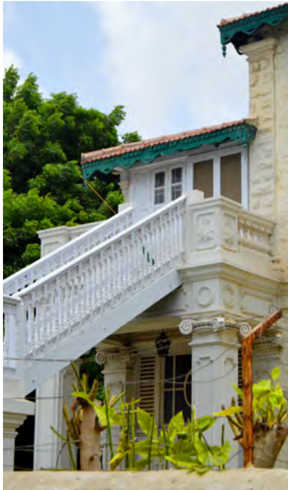
Outdoor staircase leading to first floor Image Copyright of Marvi Mazhar and Associates
