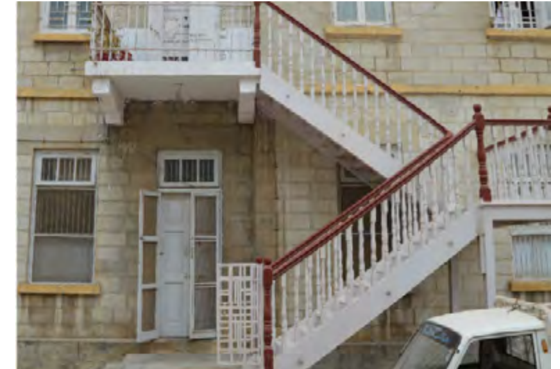
Top: Outdoor Staircase addition / Centre: Added shading device on roof level / Bottom: Wooden Staircase, railing and wooden divider with four glass panes Image Copyright of Marvi Mazhar and Associates
