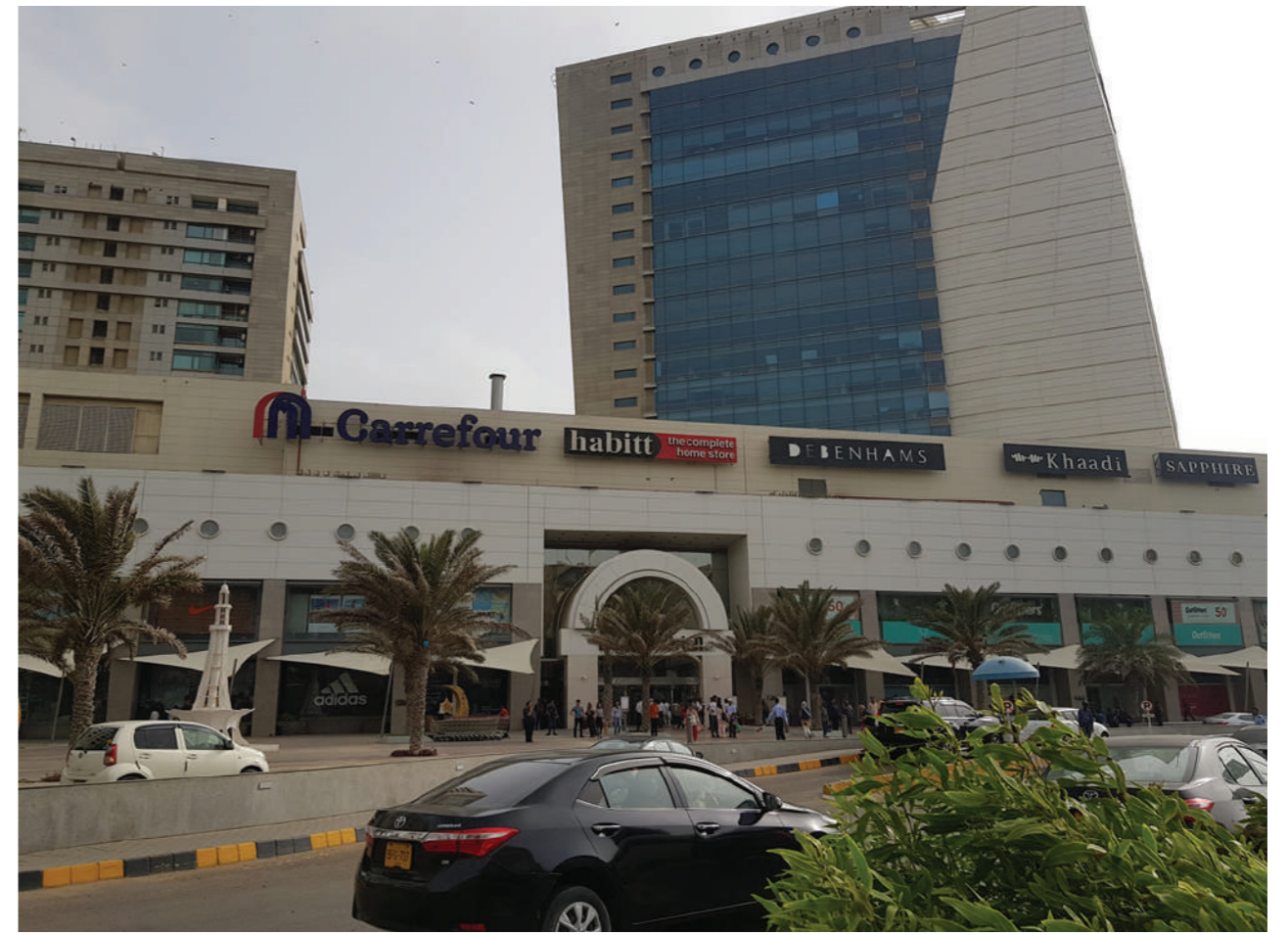
North Elevation of Dolmen Mall
