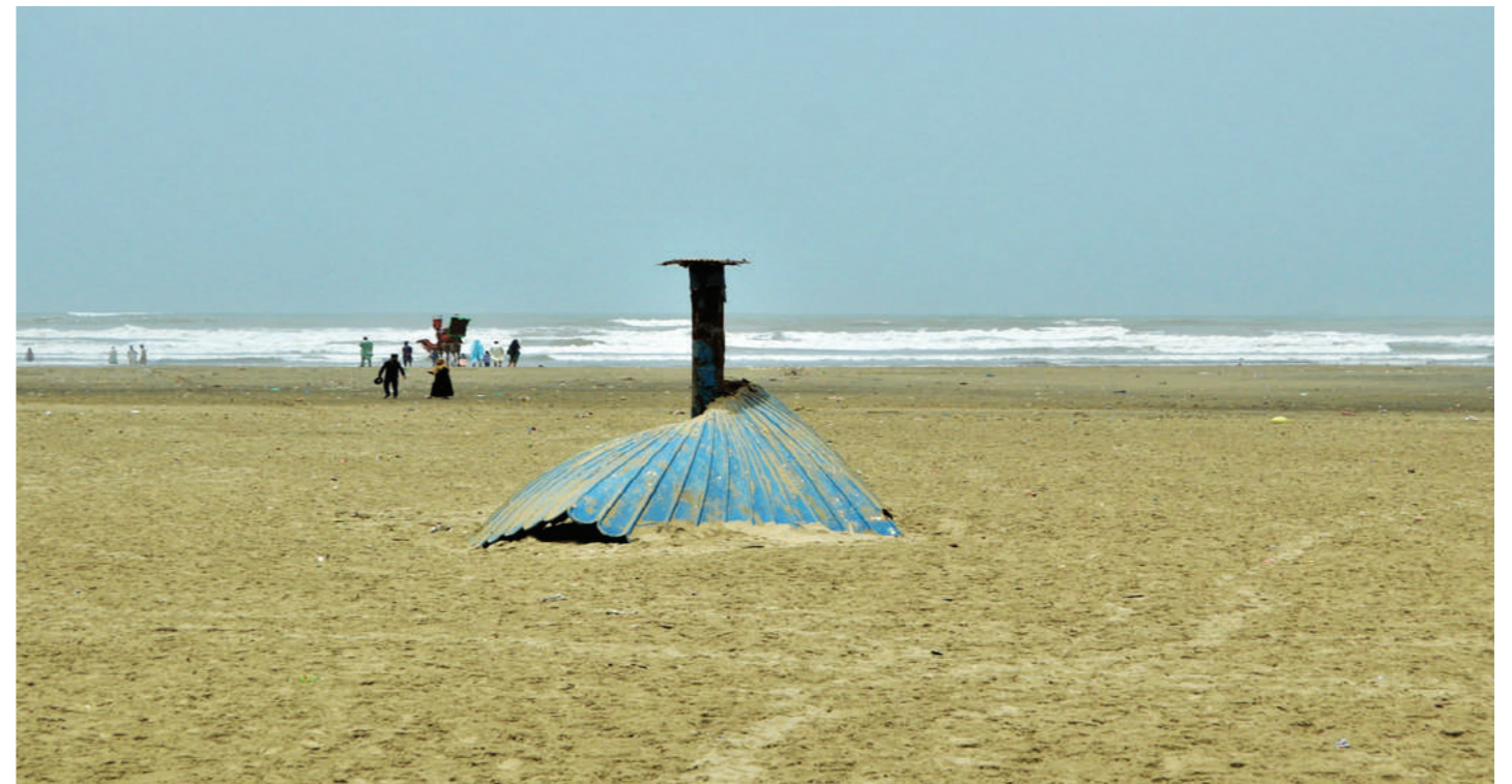
Although the umbrella's steel base is firm enough to withstand Karachi's weather, the plastic material has disintegrated.
