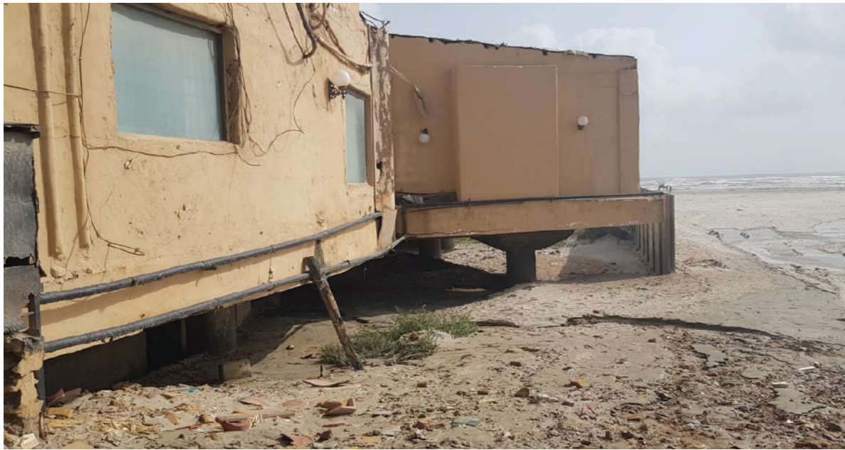
The pilotis raise the structure
