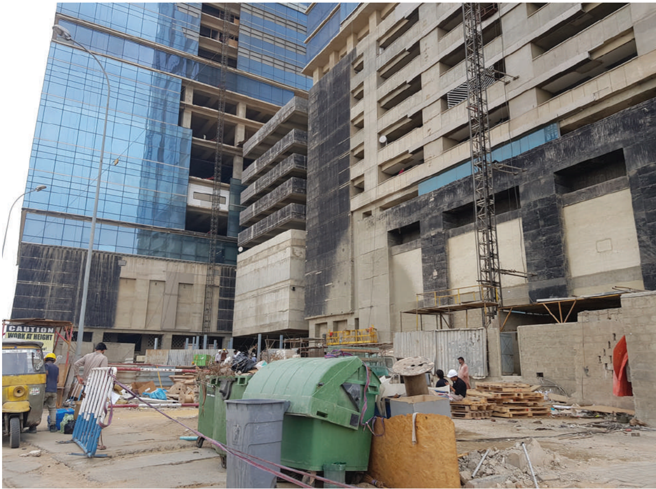
Ongoing construction on complex
