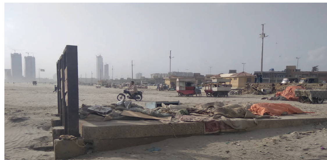
Pier being utilized as resting surface
