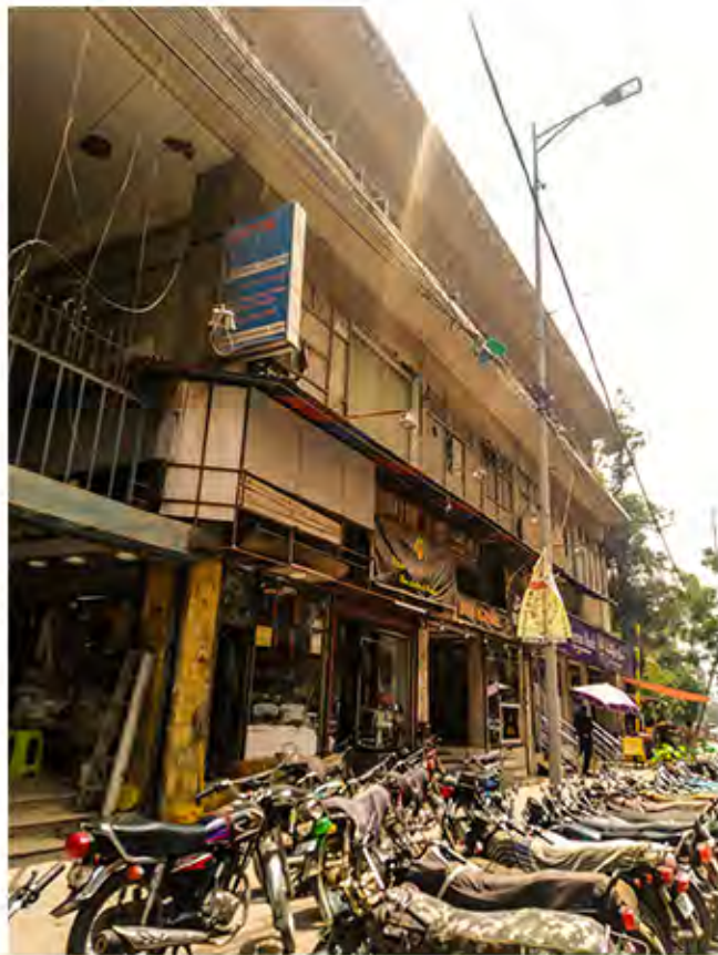
The picture shows the exterior of the Panorama Market building.
