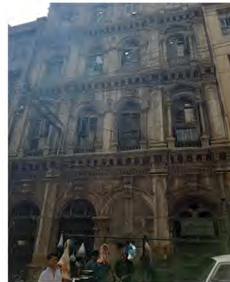
One of the many old buildings present in the bazaar.
