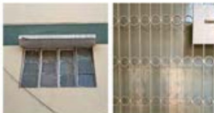
Typical Window and Grill
