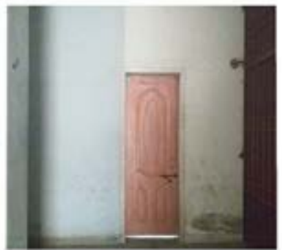
Apartments- Main Door
