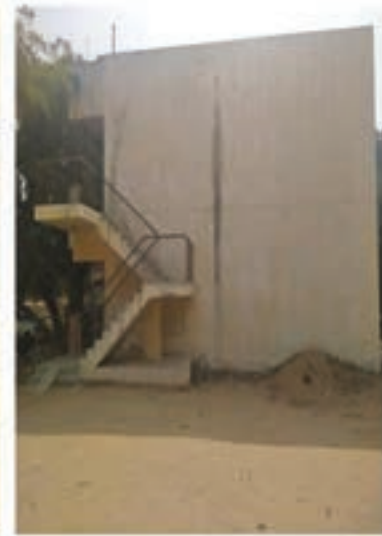
Outside StairCase On Right Side
