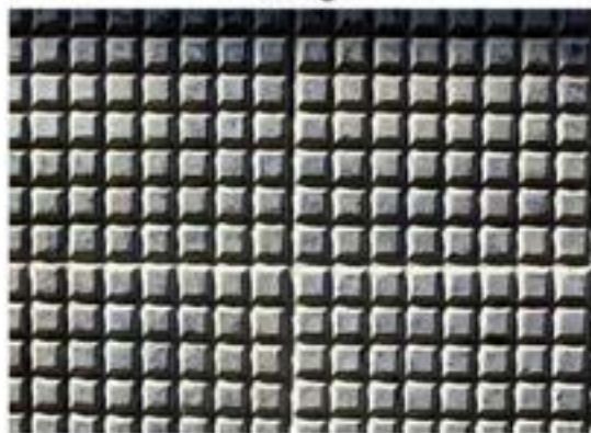
Concrete Floor Pavement
