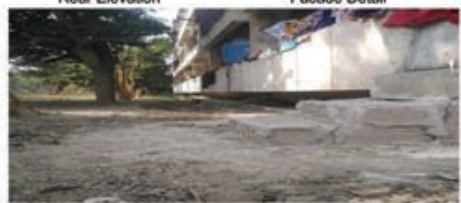
Corridor At Rear Side 2 ft. Upto thr Ground
