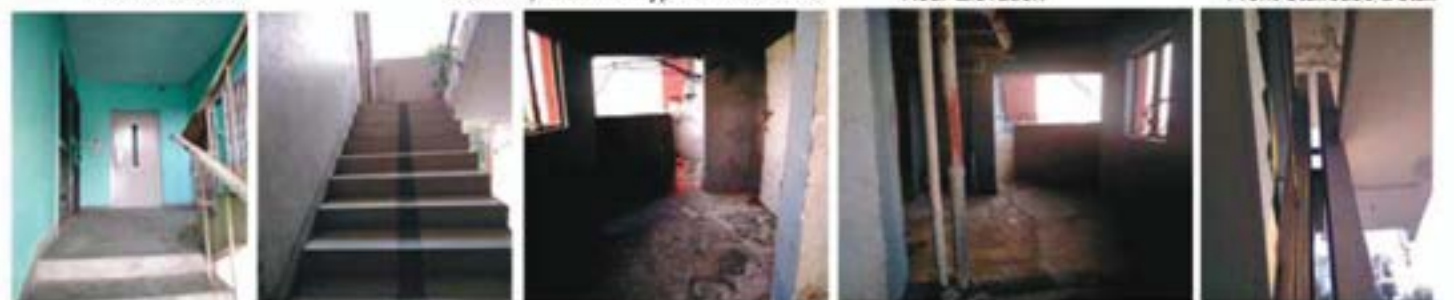
Entrance From Rear Side
