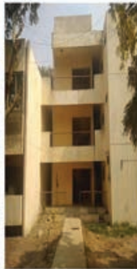
Rear Side Staircase
