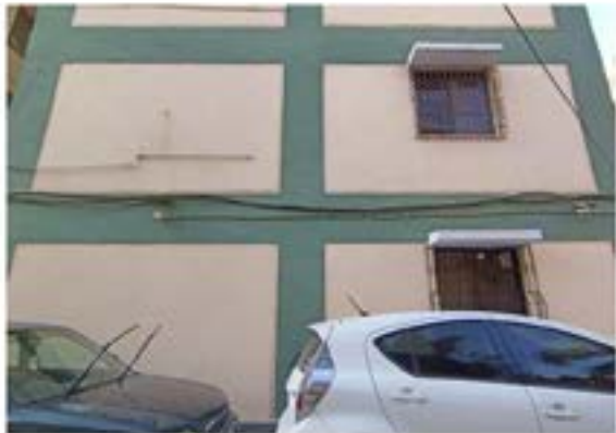
Prominent Columns and Beams
