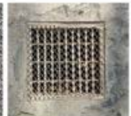
Storm Water Drain
