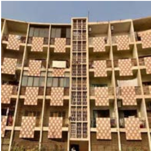
Picture by Syed Asad Ul Hasan, 2021 Screens of Island Apartments
