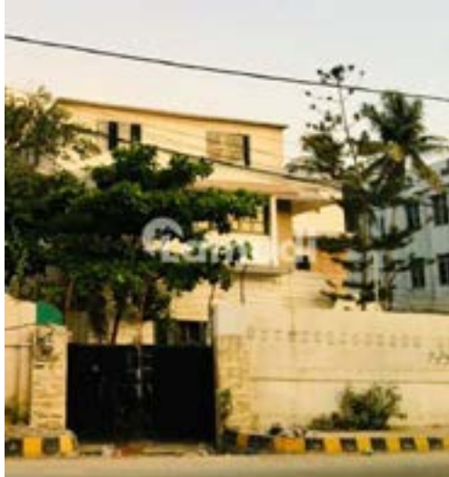
A well maintained house Jamshed Town - PECHS Block 2 (Photo credits: Lamudi.pk)
