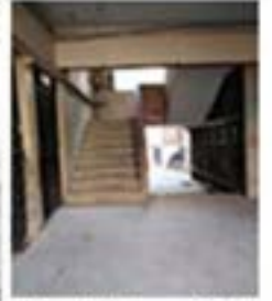
Front Staircase Detail
