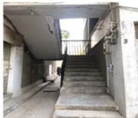
Narrow access from staircase
