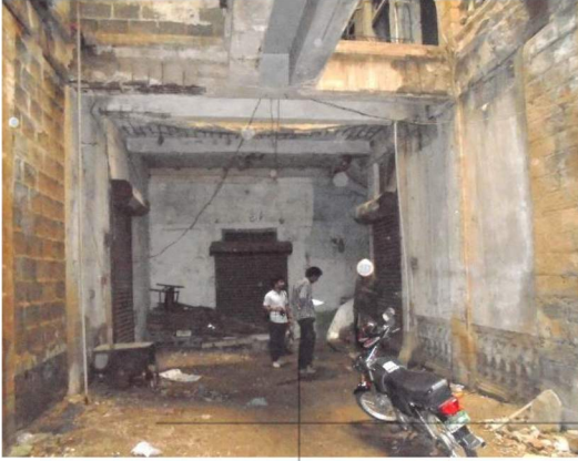
Figure 18- Students assessing the building
